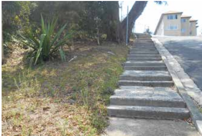
Figure 62. Steep, stepped path along Bayview Hill Road, adjacent to Forsyth Park.
