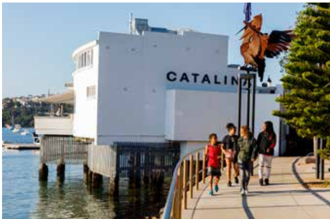
Figure 83. Site opportunities at Lyne Park include the foreshore path which is part of the Bondi to Manly walk and Harbour viewing
