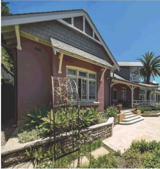
Figure 3.13 Looking north to the original house. Source: Images For Business, 2020.
