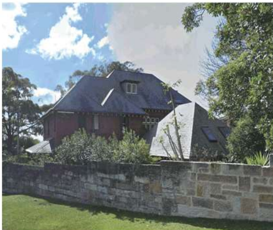
Figure 4.9 Glasson House at 19 Wentworth Road, Vaucluse. Source: Google Map
