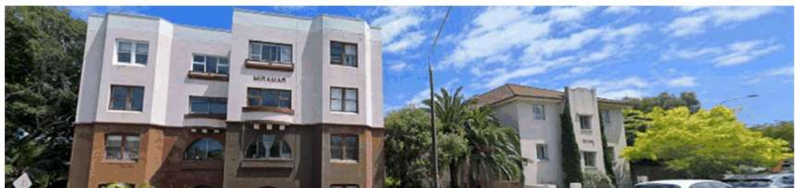
East elevation on Caledonian Rd (top) and North elevation on New South Head Rd (lower) (Source: Google Maps 2021).
