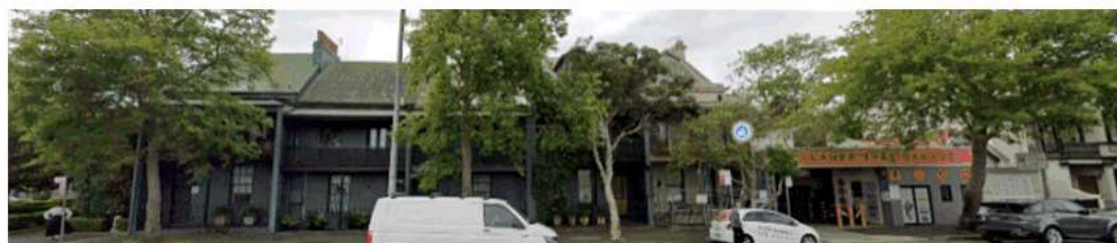
North elevation of 38-48 Oxford St (Source: Google Maps 2020).
