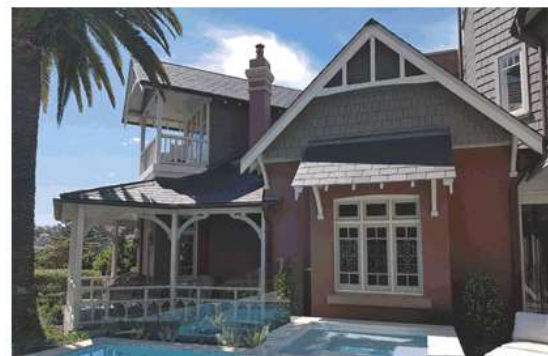
Figure 3.11 Looking south to the original house.
