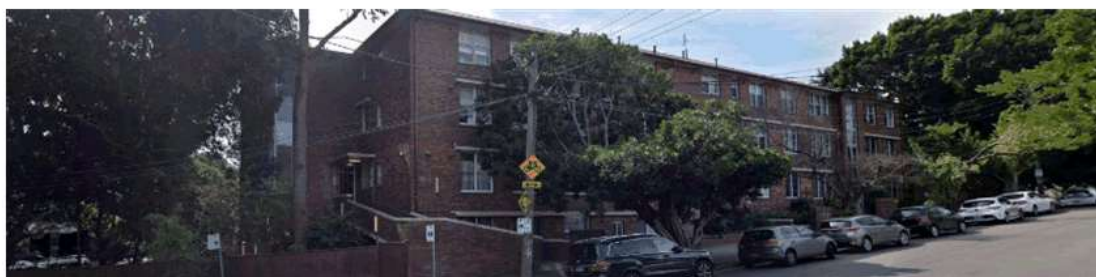
North elevation of 25 Lawson St (Source: Google Maps 2021)
