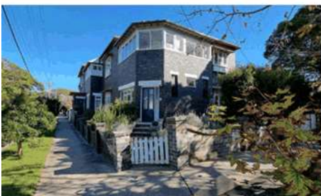
Existing Inter-War residential flat building within the study area
