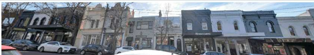
North elevation of 88 – 108 Queen St, Woollahra (Source: Google Maps 2020).
