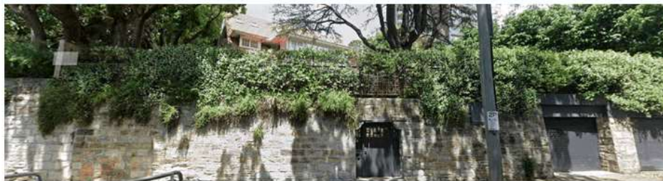
South elevation, 438 Edgecliff Rd, Edgecliff (Source: Google Maps 2021).
