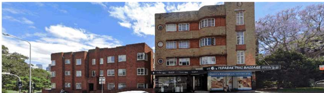
North elevation of 2-14 & 20 NSH Rd (Source: Google Maps 2021).
