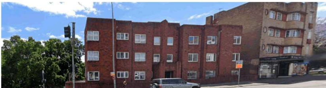
North elevation of 2-14 New South Head Rd (Source: Google Maps 2021).
