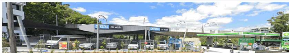
South elevation of Crystal Car Wash, 81-83 New South Head Rd, Edgecliff (Source: Google Maps 2020).
