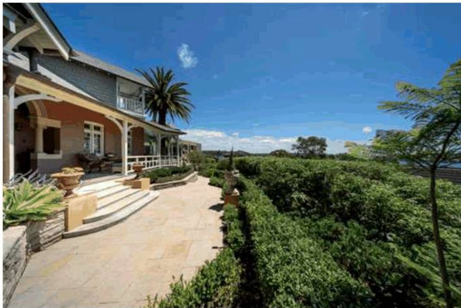
Figure 4: Looking north, showing the original house on the left and the landscape/garden in front of the house (Source: Images For Business, 2020)
