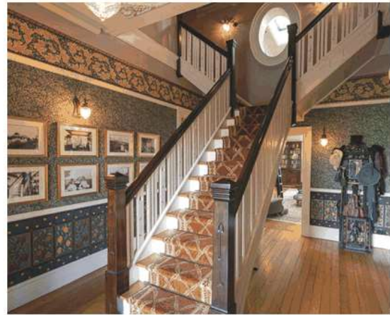
Figure 3.39 Stairs leading to the first floor, 2020. Source: Images For Business, 2020.
