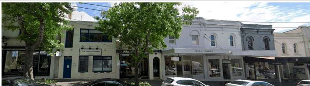
North elevation of 96 – 108 Queen St, Woollahra (Source: Google Maps 2021).
