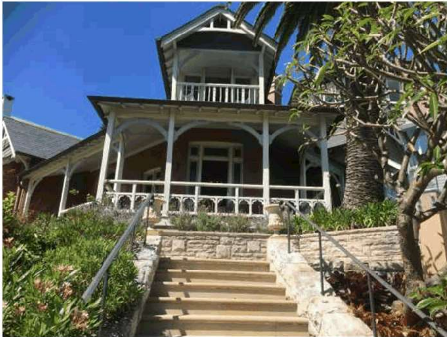
Figure 3: The original house from the entry path
