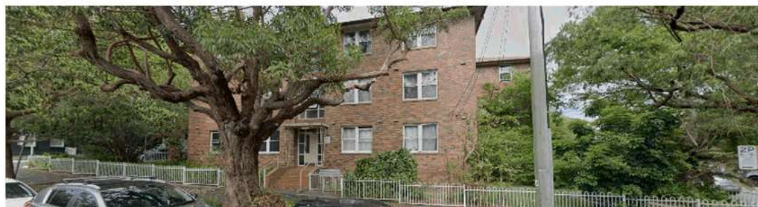
West elevation of 30 – 36 Moncur St (Source: Google Maps 2021).
