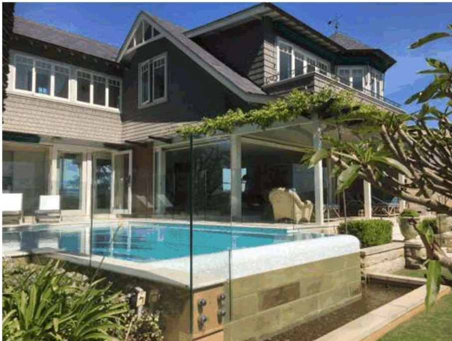
Figure 6: Front elevation of the contemporary additions
