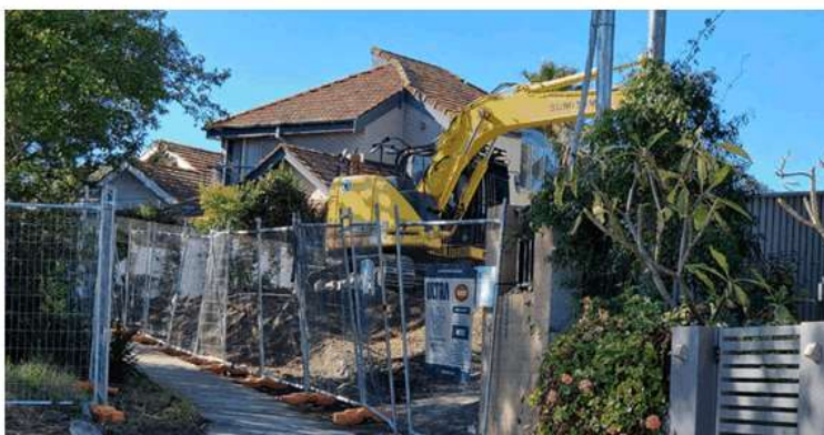
Lots currently under construction within the study area
