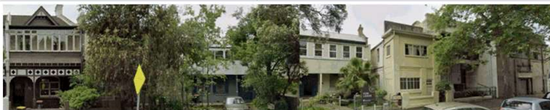
North elevation of 70 - 80 Oxford St (Source: Google Maps 2020).
