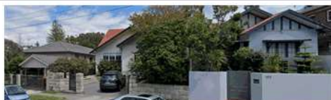
East elevation, R2 Low Density Residential on Old South Head Rd (Source: Google Maps 2021).
