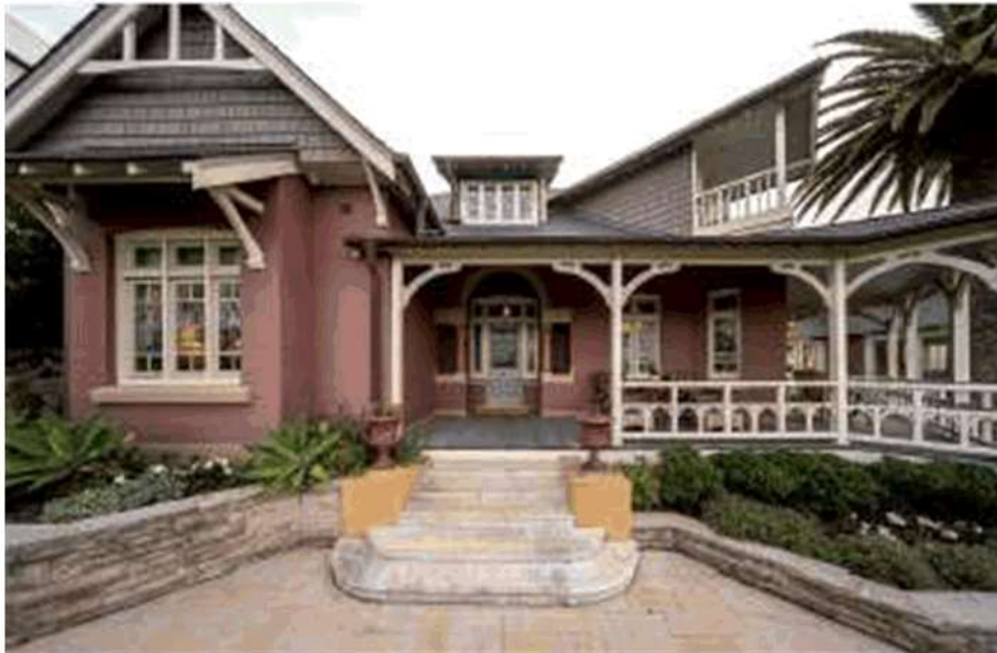
Figure 5: Front elevation of the original dwelling
