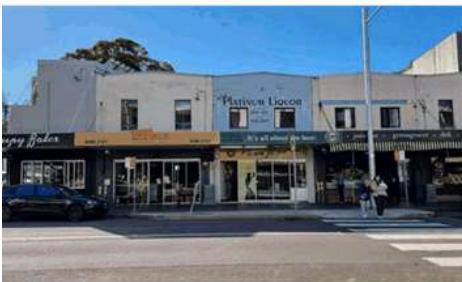
Smaller lot sizes at the intersection of Riddell Street and Bellevue Road allows for fine-grain retail
