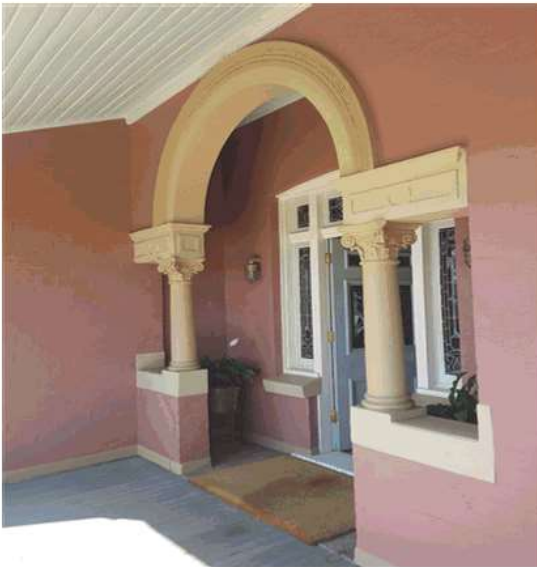
Figure 3.15 Front entrance, with original arch, columns and windows.
