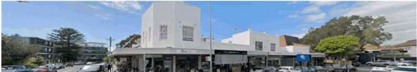
South-west elevation, B1 Neighbourhood Centre on New South Head Rd (Source: Google Maps 2021).
