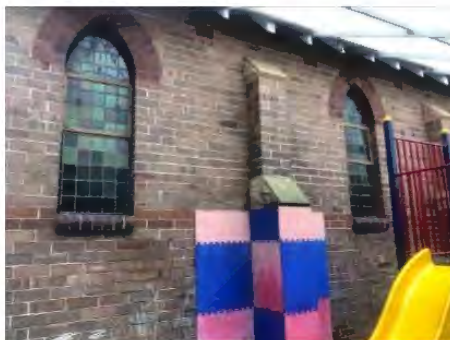
Figure 417: Detail view of leaded glass windows and piers along the side elevation of the 1909 church building.
