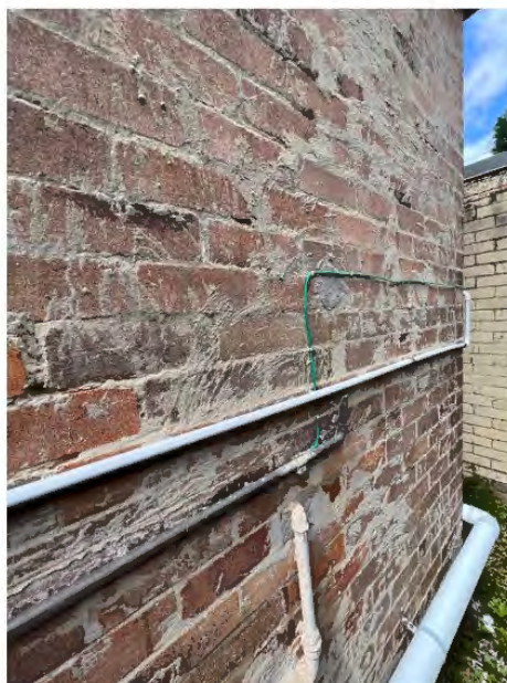
Crude mortar patching/repointing, rear wing, west elevation
