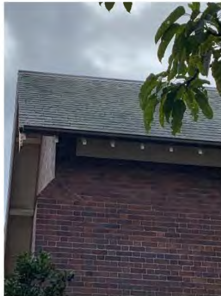
Figure 196: View of exposed rafter eaves
