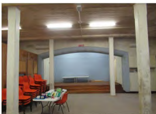
Figure 3.20 The interior of the lower ground floor of the Church of Christ building, as viewed facing south-west. Note the extensive mould on the columns and walls. Source: GBA Heritage, 19 October 2022
