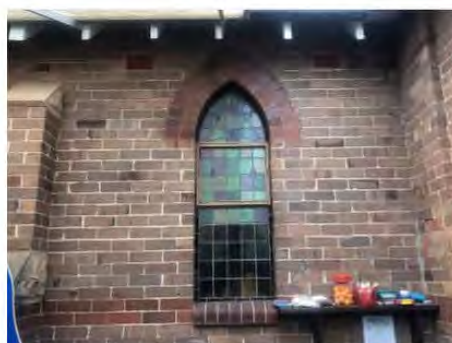
Figure 419: Detail view of leaded glass window to 1909 church building showing decorative soldier course and string course brickwork.
