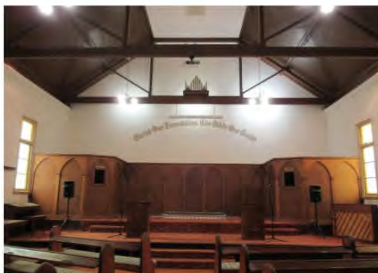
Figure 3.12 The interior of the first floor of the Church of Christ building, as viewed facing north-east. Note the timber panelled ceiling and exposed timber trusses. Source: GBA Heritage, 19 October 2022
