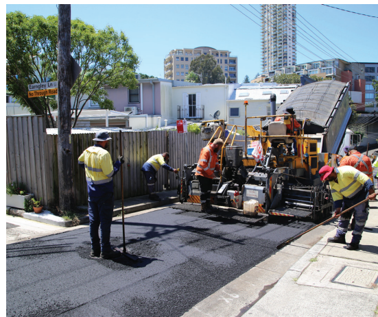
Road re-surfacing works in Edgedcliff
