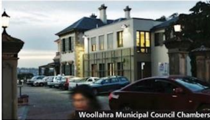
Woollahra Municipal Council Chambers
