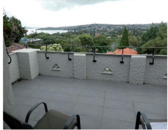
Figure 2.56 View of the upper floor balcony (originally called piazza) showing the solid decorative balustrade which was constructed later on. Note the increase the height of balustrade by the installation of steel balustrade.
