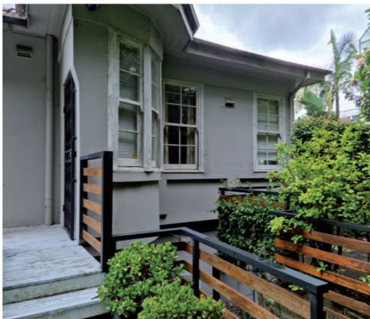
Figure 2.61 Looking to the rear (west) side of the building. Note the enclosed original piazza and its change to a bedroom. A semi-circular addition is connecting the bedroom to the balcony. A bridge is connecting the balcony to the upper garden.
