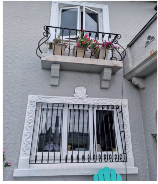
Figure 2.58 Looking to the front facade of the building. Note changes in the window frames. On the ground floor level, the window frame has a decorative architrave which is not a feature of the Spanish Mission style. Note also security screen, new Juliet balcony for the upper floor bedroom which are not representative of the Spanish Mission style.
