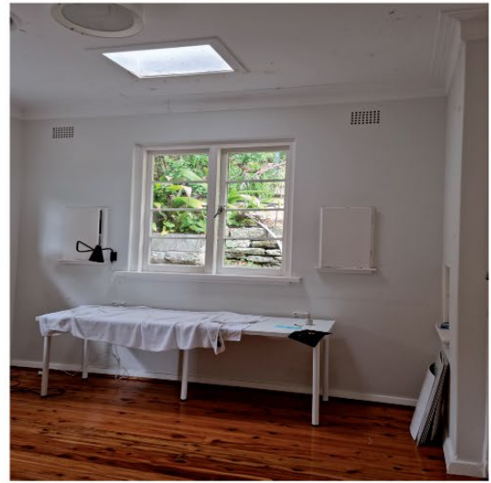
Figure 2.70 The original breakfast room. The skylight appears to have been installed later. The original window on the right hand has been bricked up.
