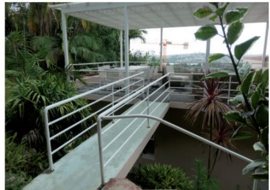
Figure 2.67 Looking to the roof terrace, showing the bridge connecting the upper level garden to the roof terrace. Note the roof terrace is covered with a steel structure and translucent glazing. The pipe railing has been replaced and the bridge was painted.
