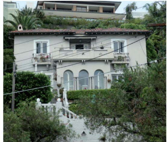
Figure 2.50 The main elevation of the building. Note extensive changes to the front facade through adding elements which are not contributing to the Spanish Mission style.
