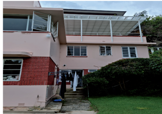
Figure 2.55 Looking to the north wing of the building, which was originally Maids' rooms. Windows were replaced on this side on the upper floor level, and a window was provided for the laundry on the ground level. The roof terrace is covered by a steel structure and translucent roof sheeting.
