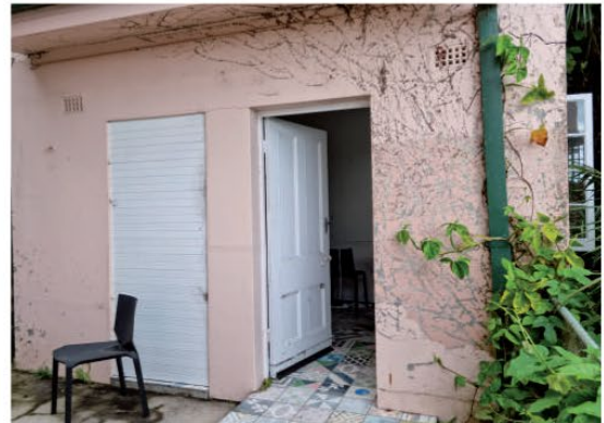
Figure 2.65 Looking to the out house on the north side of the building. This structure has undergone extensive changes over time. The original window converted to a door which is currently filled. It was originally one room which was later divided into two rooms by a partition wall. This wall was demolished.
