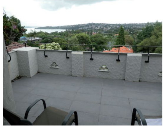
Figure 2.43 View of the upper floor balcony (originally called piazza) showing the solid decorative balustrade which was constructed later on. Note the increase the height of balustrade by the installation of steel balustrade.
