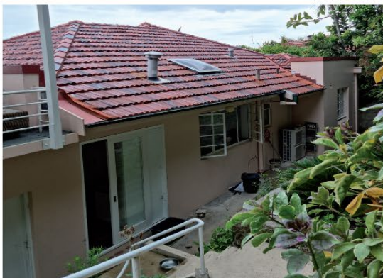
Figure 2.59 Looking to the rear (west side) of the building, showing changes to the original openings, and the installation of skylight on the roof.
