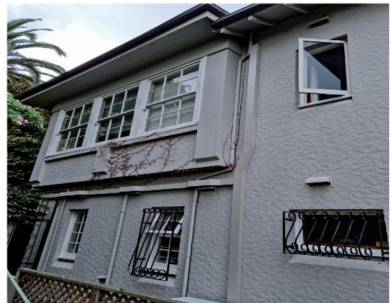
Figure 2.51 Looking to the south side of the building, showing all changes to the building including the enclosed balcony on the upper floor level.
