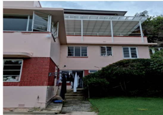
Figure 2.62 Looking to the north wing of the building, which was originally Maids' rooms. Windows were replaced on this side on the upper floor level, and a window was provided for the laundry on the ground level. The roof terrace is covered by a steel structure and translucent roof sheeting.
