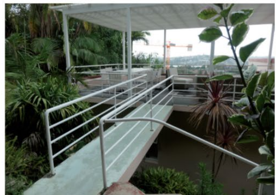
Figure 2.60 Looking to the roof terrace, showing the bridge connecting the upper level garden to the roof terrace. Note the roof terrace is covered with a steel structure and translucent glazing. The pipe railing has been replaced and the bridge was painted.
