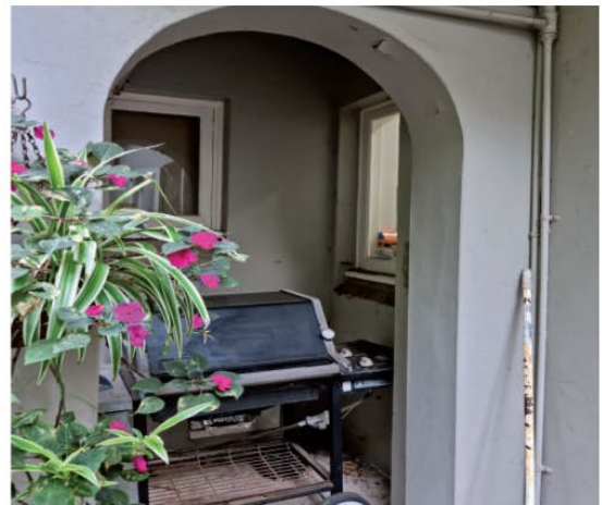
Figure 2.62 The original patio that has undergone changes. The original door from the kitchen to this space has been closed and converted to a window.
