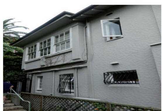
Figure 2.54 The side (south) elevation of the building, showing extensive changes to the original building including the enclosed balcony, removal of chimney stack, and changes in openings.
