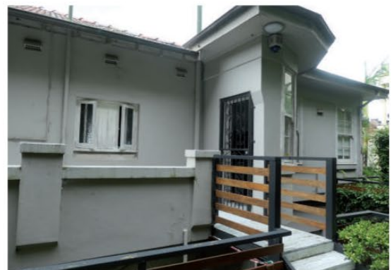
Figure 2.52 View of the rear elevation. Note extensive changes to this side of the building including enclosed balcony, construction of semicircular addition to the new bedroom, construction of a new balcony, and changes in the window frames.
