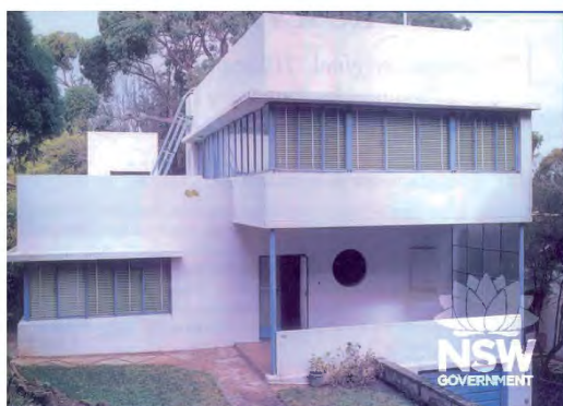
Figure 2.46 Hillman House designed by Dr Henry Epstein, 1948. Source: NSW Heritage Inventory
