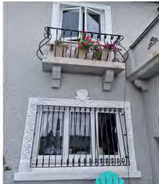
Figure 2.45 Looking to the front facade of the building. Note changes in the window frames in comparison with the original plans, security screen, new balcony for the upper floor balcony with wrought iron balustrade.
