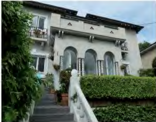
Figure 2.42 Looking to the front (main) facade of the building. Note the enclosed arched loggia, new balconies for two bedrooms on either side of the building, decorative solid balustrade for the upper floor balcony, new window frames, and security screens on the lower level floor windows.
