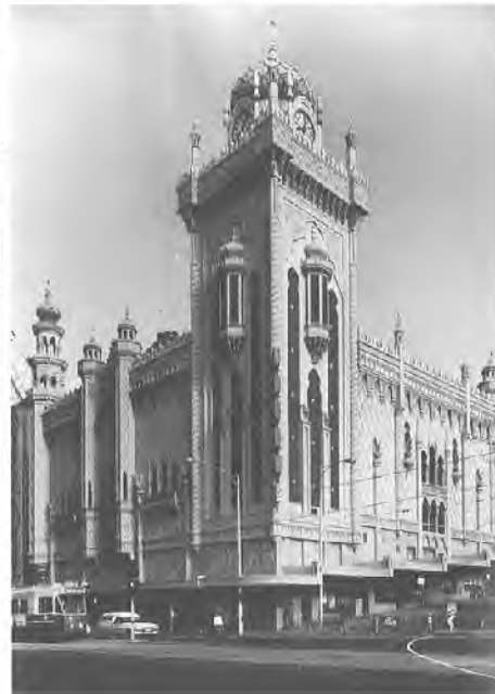
Figure 15: State Theatre, Melbourne, 1929. Architects: Bohringer, Taylor & Johnson (Source: Apperly, Irving & Reynolds, 1989, Identifying Australian Architecture , p.176).
