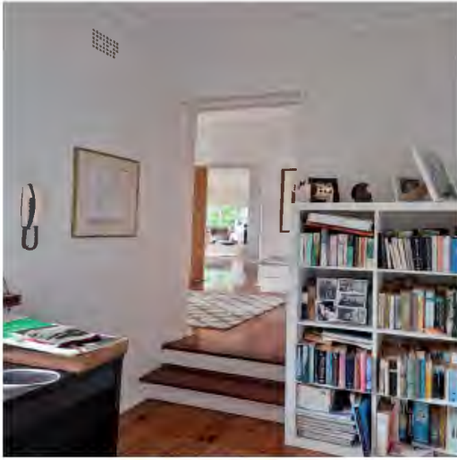
Figure 2.69 The original maid's room that converted to a study room for the bedroom. Note two stairs that appear to have been constructed recently.
