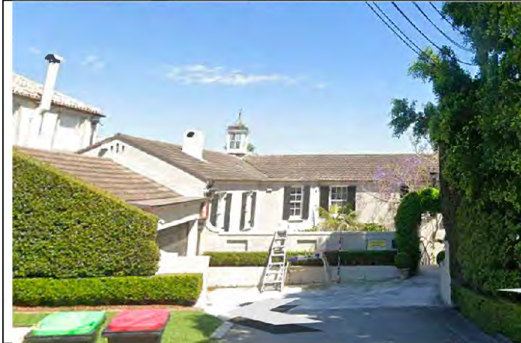
Figure 8.18: 1969: 20 The Crescent, Vaucluse. Architect: Leslie Wilkinson (Source: Google Earth Pro, accessed 8 February 2022)
