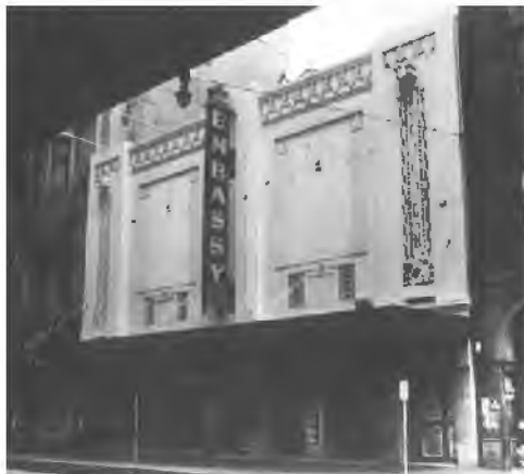
Figure 16: Embassy Theatre, Sydney, 1934. Architects: Bohringer, Taylor & Johnson (Source: Ross Thorne, 1984, Cinemas of Australia via USA , p.140).
