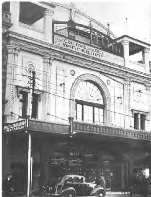
Figure 14: Regent Theatre, Melbourne, 1927. Architects: Bohringer, Taylor & Johnson (Source: Ross Thorne, 1984, Cinemas of Australia via USA , p.306).
