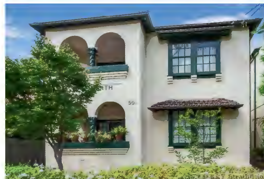
Figure 2.14 Two storey Spanish Mission style building at 50A Wentworth Road. Source: https://www.realestate.com.au/property/unit-1-50a-wentworth-rd-burwood-nsw-2134
