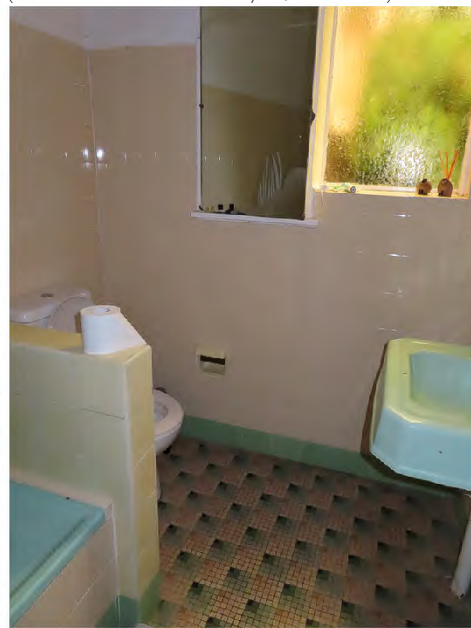
Figure 7.32: Original bathroom in lower level. (Source: Robertson & Hindmarsh Pty Ltd, 1 March 2022)
