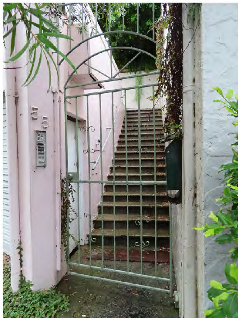
Figure 7.9: Entry gate and stairs to garage roof from the street. (Source: Robertson & Hindmarsh Pty Ltd, 1 March 2022)
