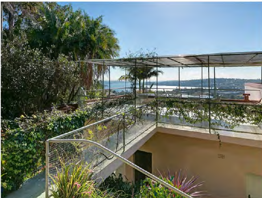
Figure 23: 55 Drumalbyn Road, Bellevue Hill, original roof terrace and access bridge from the upper garden level. Note the original pipe handrail (extant) and the pipe pergola (since replaced). Architect: P. Gordon Craig & John M. Brindley, 1937 (Source: realestate.com.au – accessed 3/12/21)
