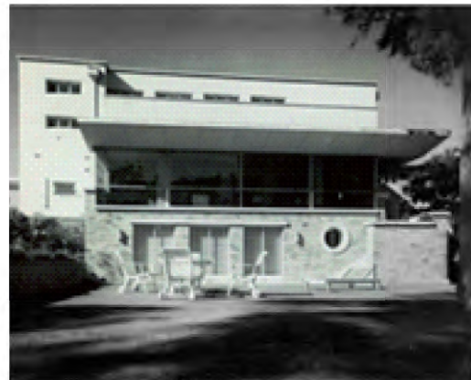
Figure 2.45 Eisner House in Warrawee designed by H. Stossel in c.1947. It is demolished. Source: Sydney Living Museum.
