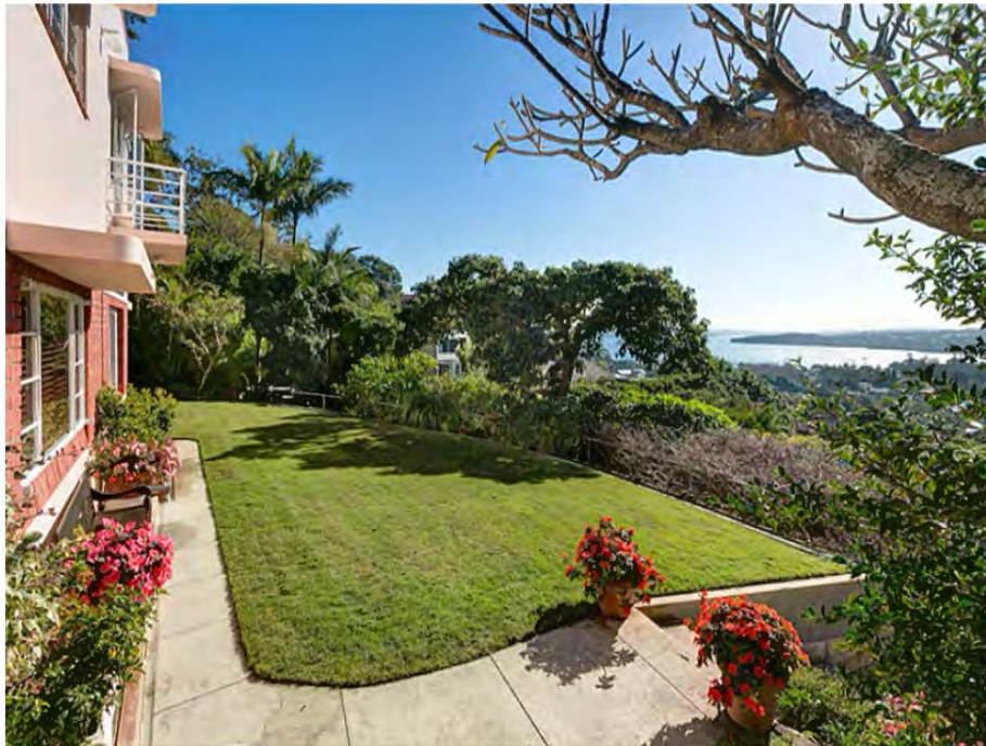
Figure 21: 55 Drumalbyn Road, Bellevue Hill, front yard with panoramic views. Note the render and brick façade treatment, the cantilevered balcony with pipe handrail, concrete hoods over the windows and the original wall light fitting. Architect: P. Gordon Craig & John M. Brindley, 1937 (Source: realestate.com.au – accessed 3/12/21)
