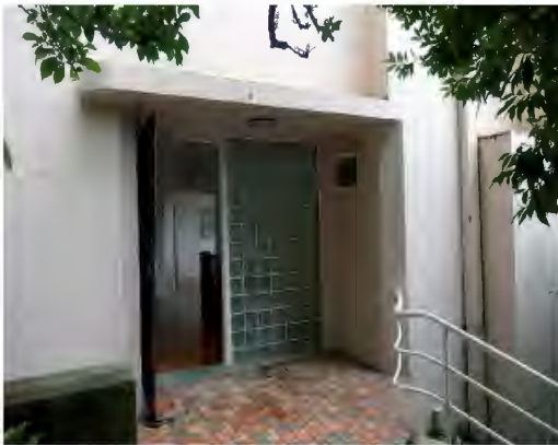
Figure 2.63 Entrance to the building on the south side.
