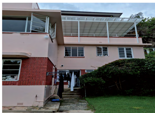
Figure 2.55 Looking to the north wing of the building, which was originally Maids' rooms. Windows were replaced on this side on the upper floor level, and a window was provided for the laundry on the ground level. The roof terrace is covered by a steel structure and translucent roof sheeting.
