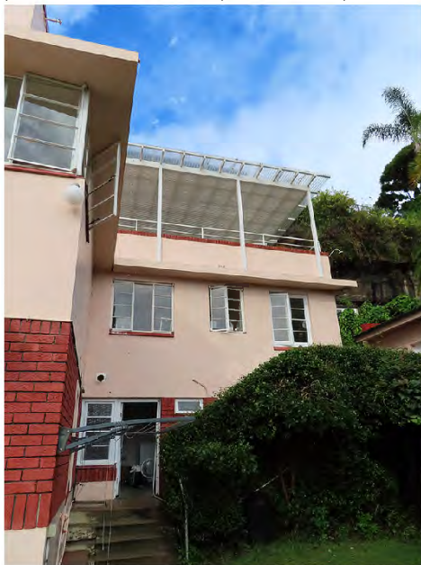
Figure 7.15: Looking south at the front façade of the west wing. (Source: Robertson & Hindmarsh Pty Ltd, 1 March 2022)
