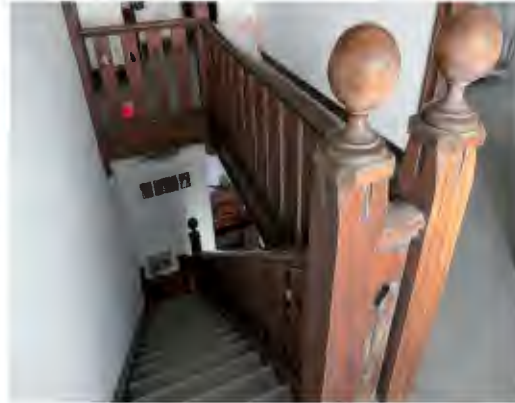
Figure 2.59 View of the staircase leading up to the upper floor level.
