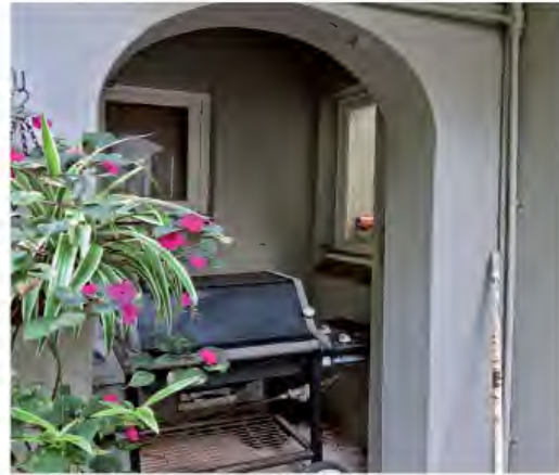
Figure 2.49 The original patio that has undergone changes. The original door from the kitchen to this space has been closed and converted to a window.
