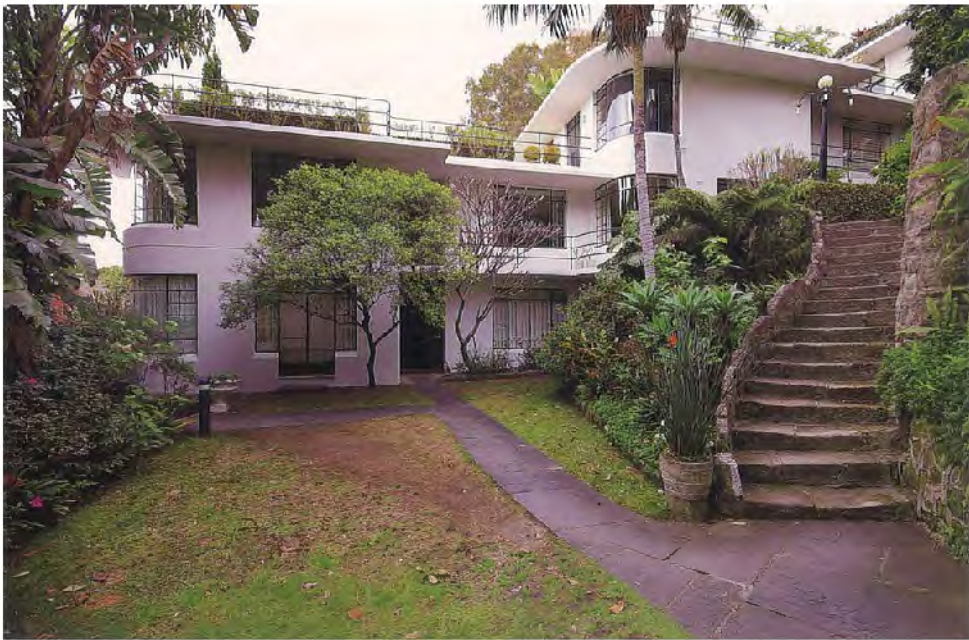
Figure 8.14: "Wyldefel Gardens", Potts Point, Sydney. Architect: John Brogan, 1936 (Source: Lewi & Goad, 2019, Australian Modern , p.42)
