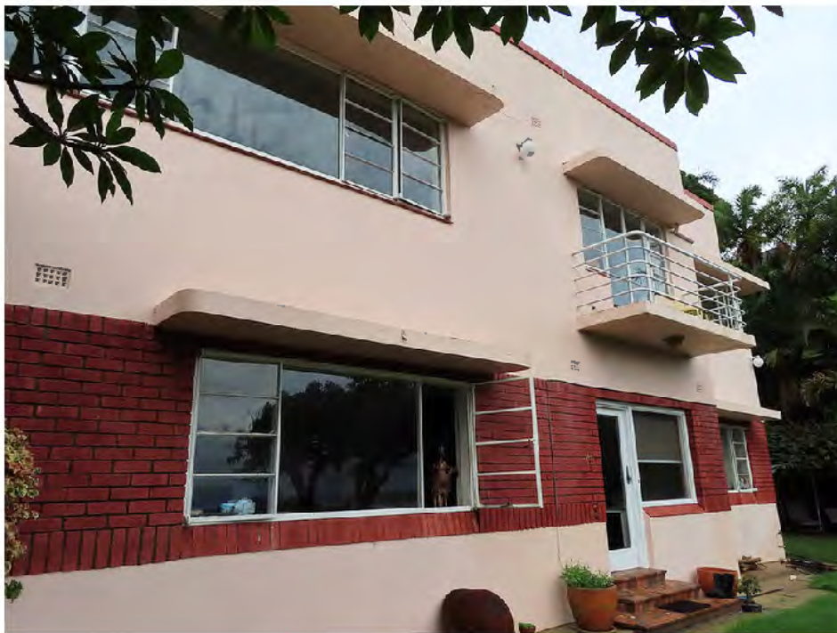
Figure 7.4: 55 Drumalbyn Road, Bellevue Hill, front façade. Note the render and brick façade treatment, the cantilevered balcony with pipe handrail, concrete hoods over the windows, the original wall light fitting, and the original soffit light fitting under the balcony. Architect: P. Gordon Craig & John M. Brindley, 1937. (Source: Robertson & Hindmarsh Pty Ltd, 1 March 2022)
