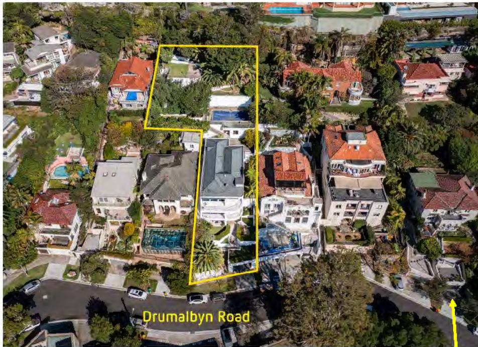
Figure 5.24: June 2021. An aerial view of the western side of Drumalbyn Road. No. 53 is indicated with an arrow. (Source: realestate.com.au: Laing+Simmons – Double Bay, 63-65 Drumalbyn Road Bellevue Hill, June 2021)
