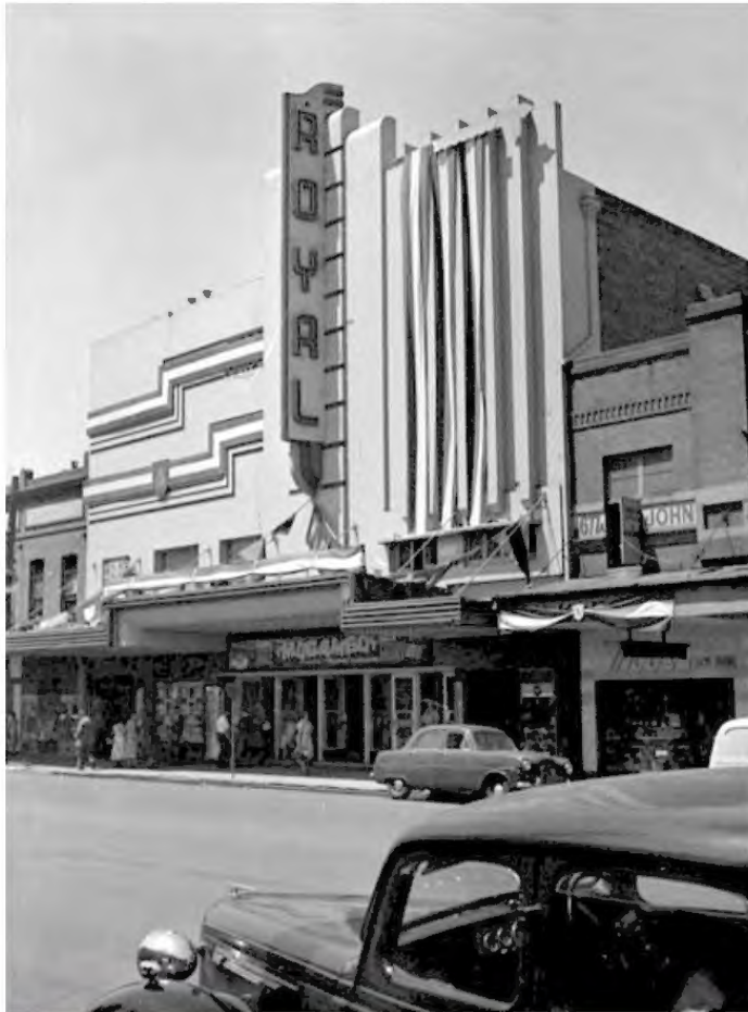
Figure 6.44: Theatre Royal, Newcastle, 1938 (an Art Deco makeover of a 1924 theatre designed by Charles Bohringer). Architect: Charles Bohringer (Source: Cinema Treasures, cinematreasures.org, accessed 12 January 2022).
