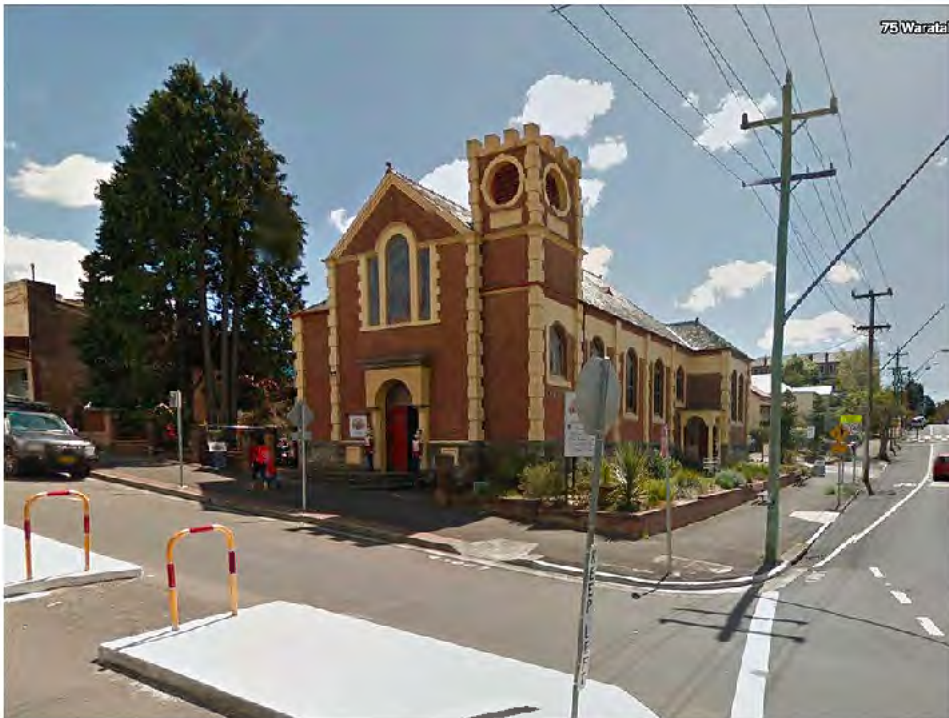
Figure 6.1: St Andrew's Presbyterian Church, Waratah & Lurline Streets, Katoomba, 1913-1914. Architect: P. Gordon Craig (Source: Google Earth Pro, accessed 24 December 2021)
