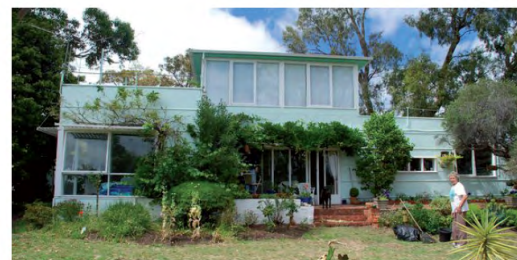
Figure 2.20 The Ship, designed by Roy Grounds as his residence, in c.1934. Source: https://vhd.heritagecouncil.vic.gov.au
