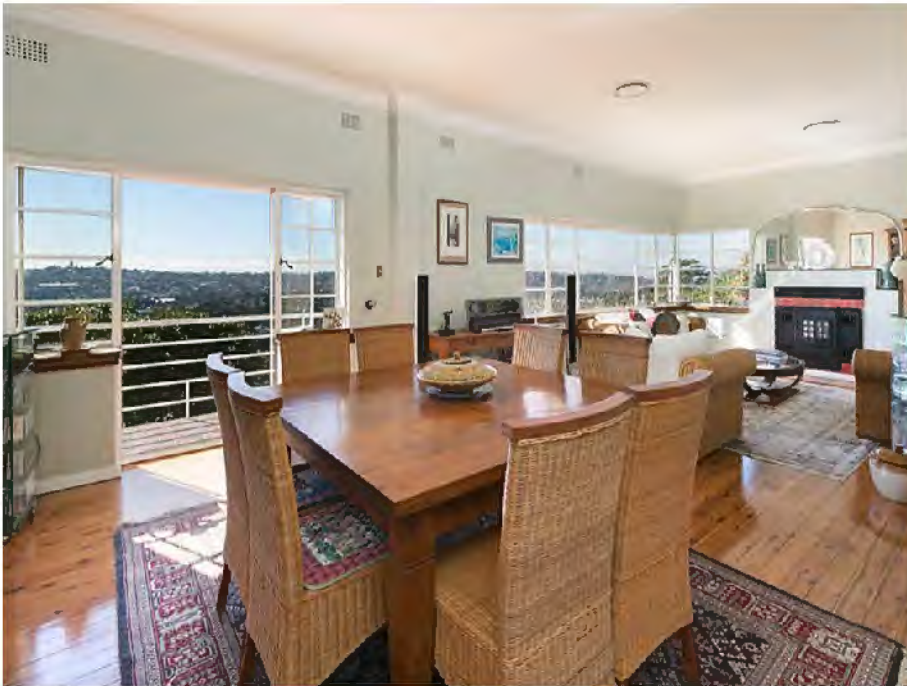
Figure 22: 55 Drumalbyn Road, Bellevue Hill, Living/Dining Room with horizontal strip steel-framed corner windows and steel door and window set leading to the balcony. Architect: P. Gordon Craig & John M. Brindley, 1937 (Source: realestate.com.au – accessed 3/12/21)
