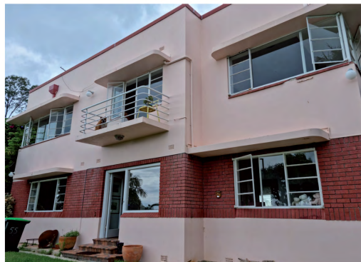
Figure 2.54 Looking to the front (main) facade of the building, showing architectural features of the style.
