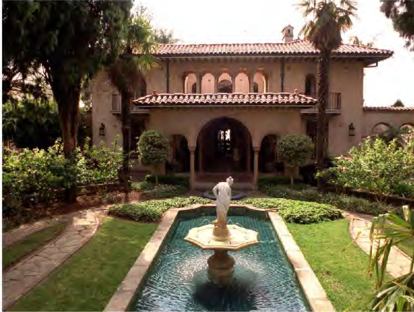
Figure 11: Entry porte cochere/loggia, "Boomerang", Billyard Avenue, Elizabeth Bay. Architect: Neville Hampson, 1926 (Source: realestate.com.au – accessed 9/12/21)
