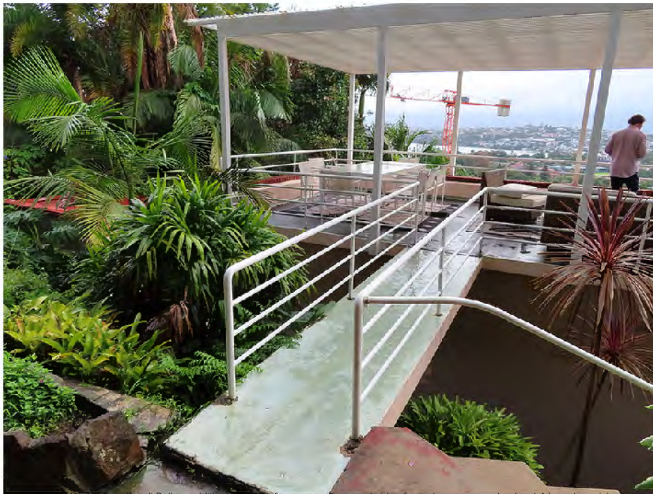
Figure 7.6: 55 Drumalbyn Road, Bellevue Hill, original roof terrace and access bridge from the upper garden level. Note the original pipe handrail (extant) and non-original pergola. Architect: P. Gordon Craig & John M. Brindley, 1937. (Source: Robertson & Hindmarsh Pty Ltd, 1 March 2022)
