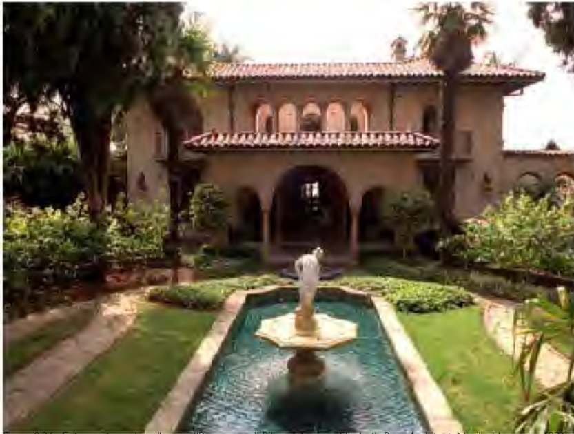
Figure 8.26: Entry porte cochere/loggia. "Boomerang," Billyard Avenue, Elizabeth Bay. Architect: Neville Hampson, 1926 (Source: realestate.com.au – accessed 9/12/21)
