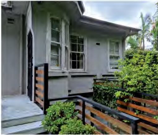
Figure 2.48 Looking to the rear (west) side of the building. Note the enclosed original piazza and its change to a bedroom. A semi-circular addition is connecting the bedroom to the balcony. A bridge is connecting the balcony to the upper garden.
