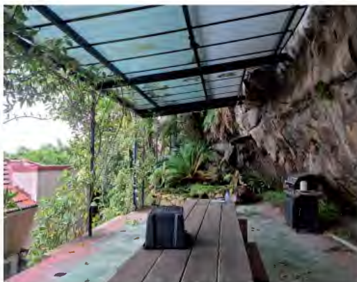
Figure 2.61 Upper level garden with steel structure and translucent glazing sheets.
