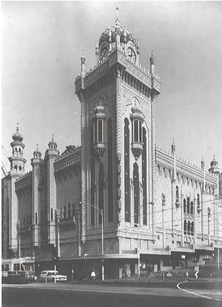
Figure 6.14: Forum (former State) Theatre, Melbourne, 1929. Architects: Bohringer, Taylor & Johnson (Source: Apperly, Irving & Reynolds, 1989, Identifying Australian Architecture , p.176).
