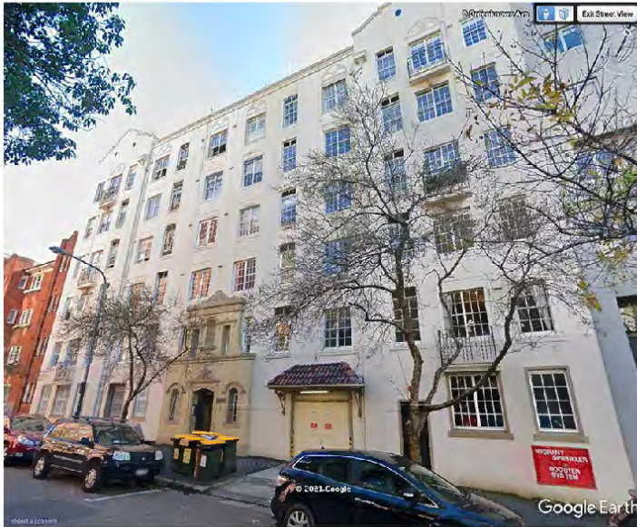
Figure 6.32: 2 Greenknowe Avenue, Elizabeth Bay; Architects: Bohringer, Taylor & Johnson, 1929 (Source: Google Earth – accessed 15 December 2021)
