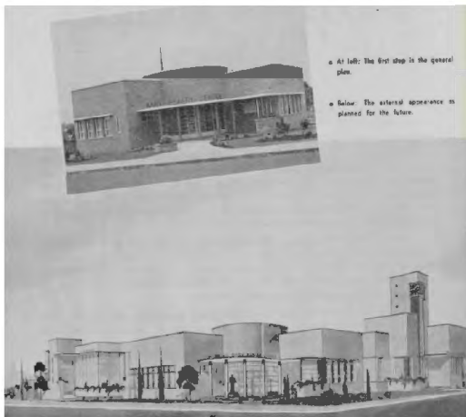
Figure 2.14 Punchbowl Health Centre designed by Davey and Brindley, displaying modern architecture style. Source: Trove, Decoration and glass magazine , January-February 1948.
