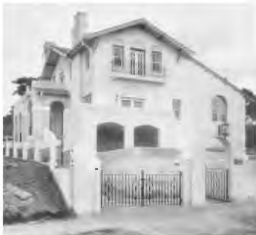
Figure 2.18 Doctor's Town House in VIC. Source: The Australian Home Builder , 1925.
