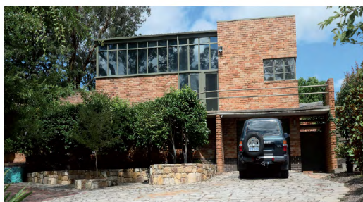
Figure 2.27 The Moir Residence at Forrest, ACT, 1935 Source: GBA Heritage , 2022.
