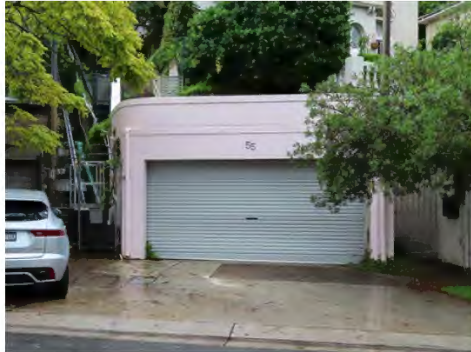
Figure 7.7: Original garage with entry gate to the right. (Source: Robertson & Hindmarsh Pty Ltd, 1 March 2022)
