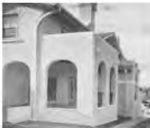
Figure 2.16 The parged or roughly trowelled cement provides a unique decorative effect which is a striking feature of Mission style exterior. Source: The Australian Home Builder , 1925.
