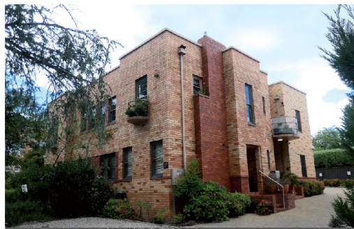
Figure 2.34 Forrest Fire Station and residences Source: GBA Heritage, 2022
