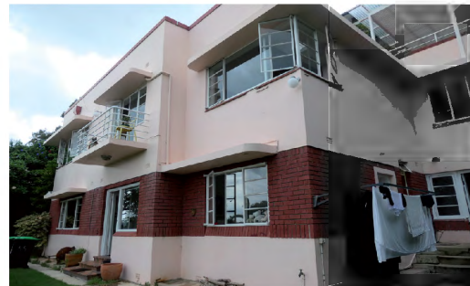
Figure 2.32 The subject house at 55 Drumalbyn Road, Bellevue Hill Source: GBA Heritage, 2022
