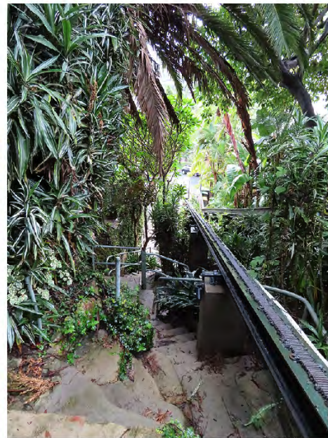
Figure 7.10: Looking down access stairs and inclinator towards the street. (Source: Robertson & Hindmarsh Pty Ltd, 1 March 2022)
