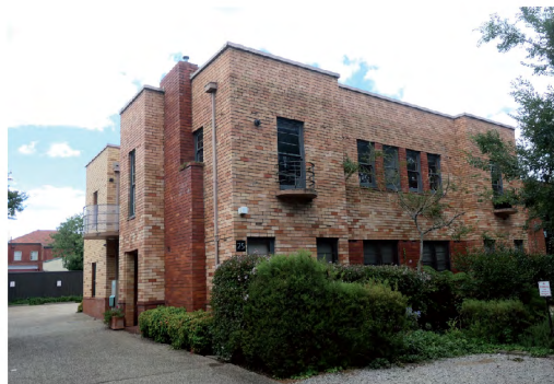
Figure 2.35 Forrest Fire Station and residences Source: GBA Heritage, 2022.
