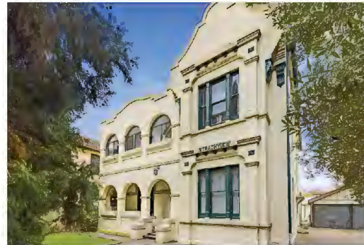
Figure 2.13 Two storey Spanish Mission style building at 50 Wentworth Road. Note the first floor level infilled arches. Source: https://www.domain.com.au/property-profile/50-wentworth-road-burwood-nsw-2134
