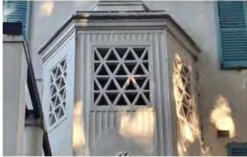
Figure 29 Spanish Mission detailing (grilled openings) for ventilation from Silchester Flat, designed by Leslie Wilkinson in 1929 at 4 Trahlee Road, Bellevue Hill
