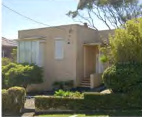
Figure 125 Front elevation of 6 Princes Avenue, Vaucluse (Source: Photo: Google streetview)
