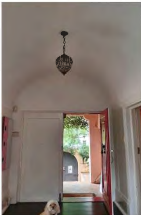
Figure 30 Vaulted ceiling in the main hallway
