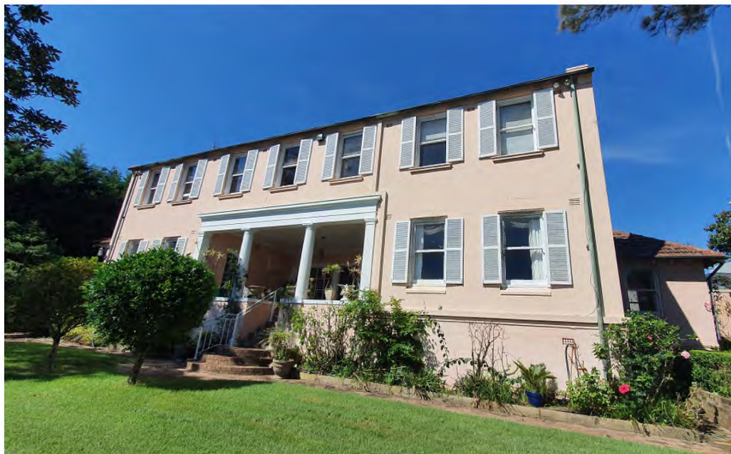
Figure 7: North facing elevation of 43 Latimer Road, Bellevue Hill with doric columns supporting an entablature
