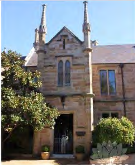
Figure 327 10 Dunara Gardens, Point Piper (Source: Photo: SHR, 2015)
