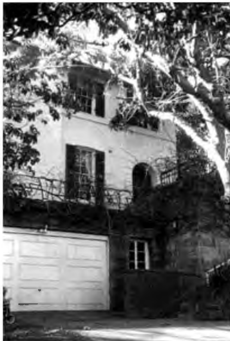
Figure 272 Photo of 5-7 Trahlee Road from the Australian Institute of Architects Register cards, No.4700698.
