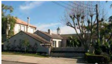
Figure 202 20 The Crescent, Vaucluse from the street
