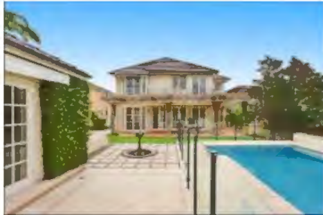
Figure 106 Rear elevation of 45 New South Head Road, Vaucluse (Source: www.realestate.com.au 2016)
