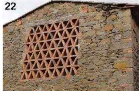
Figure 30 Vernacular grilled openings in rural building at Greve in Chianti, Firenze (Source: www.ilcapochiave.it )
