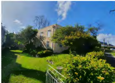
Figure 126 View of the house and its north garden from Princes Avenue, Vaucluse
