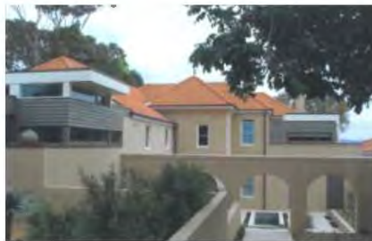
Figure 102 View from entry path after to the 2008 alterations and additions
