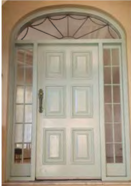
Figure 18 Front door of 45 New South Head Road, Vaucluse with fanlight and sidelights. Leslie Wilkinson designed alterations and additions to this house in 1937.
