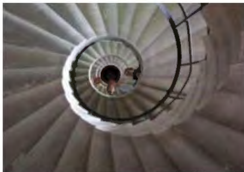
Figure 43 Helicoidal staircase of Urbino, Montefeltro Palace ( www.edilcoscale.it )
