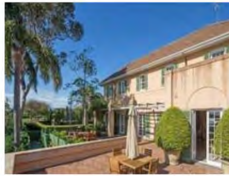
Figure 245 1 Rose Bay Avenue, Bellevue Hill north elevation (Source: www.realestate.com.au )
