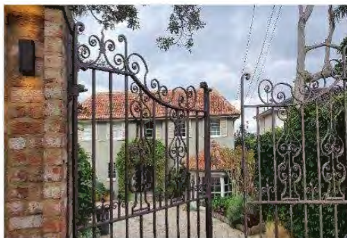
Figure 159 Detail of the wrought iron front gate by Wilkinson
