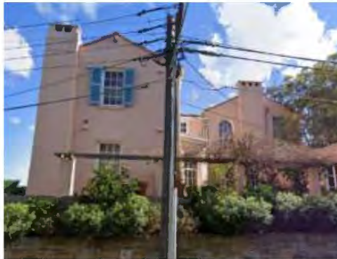
Figure 37 eastern elevation of Greenway, designed by Leslie Wilkinson as his own house in 1922.
