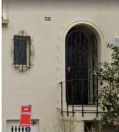
Figure 226 Wrought iron gate to 6 Wiston Gardens, Darling Point.
