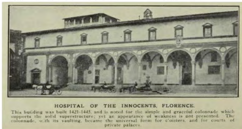
HOSPITAL OF THE INNOCENTS, FLORENCE. This building was built 1421-1445, and is noted for the simple and graceful colonnade which supports the solid superstructure; yet an appearance of weakness is not presented. The colonnade, with its vaulting, became the universal form for cloisters, and for courts of private palaces. Figure 24 Brunelleschi's Hospital of the Innocents in Florence (Source: Wilkinson, 1920b, p 72)
