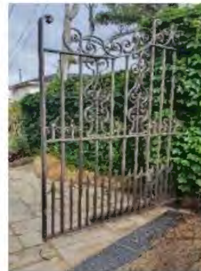
Figure 158 Detail of the wrought iron front gate by Wilkinson
