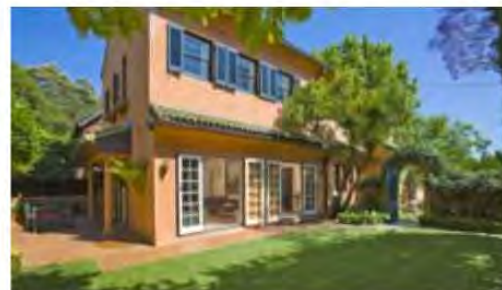
Figure 139 View of the second floor addition to the rear wing (Source: www.realestate.com.au , 2011)
