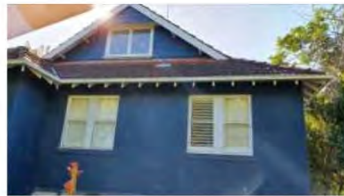
Figure 80 Rear elevation of 109 O'Sullivan Road, Bellevue Hill
