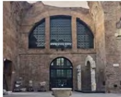
Figure 32 Diocletian window: a semi-circular arch shaped opening segmented into thirds with two vertical dividers. So called after the Diocletian Baths in Rome ( www.orizzontecultura.com )
