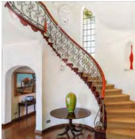
Figure 228 Wrought iron balustrade to the prominent staircase.
