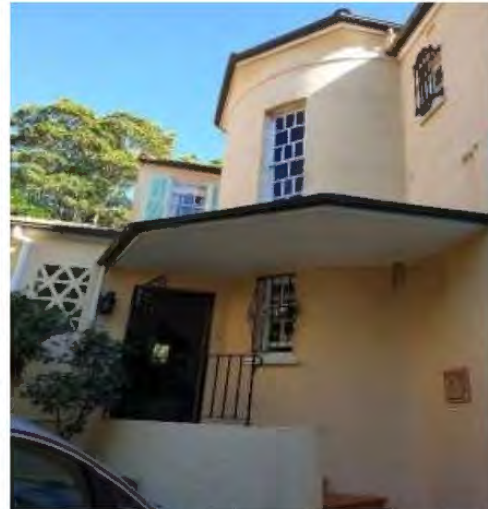
Figure 42 Entry way tower incorporating the main staircase from Leslie Wilkinson designed house at 80A Hopetoun Avenue, Vaucluse
