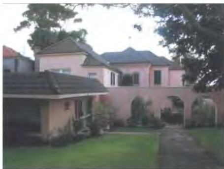
Figure 101 View from entry path prior to the 2008 alterations and additions
