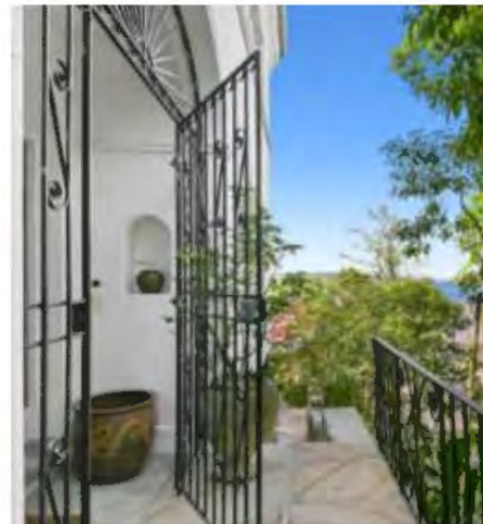
Figure 229 Wrought ironwork to 30 Wyuna Road, Point Piper.
