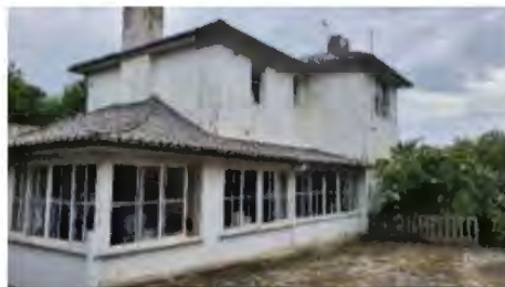
Figures 117 and Figure 118 Views to Southmoor
