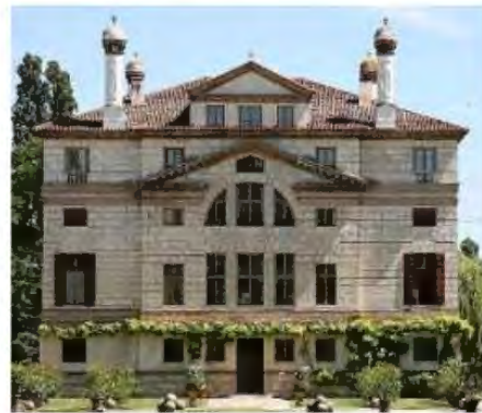
Figure 34 Another example of Diocletian or thermal window in Villa Foscari by A. Palladio (Source: WikiWand)
