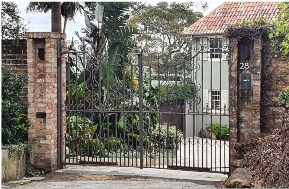
Figure 34 Wrought iron gate designed by Professor Leslie Wilkinson
