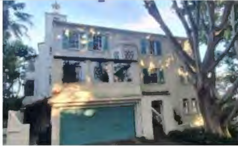
Figure 246 Silchester Flats main elevation
