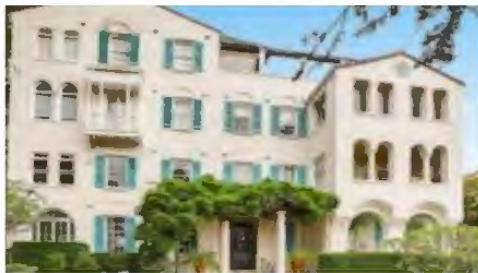
Figure 247 Silchester Flats north facing elevation (source: www.realestate.com.au )
