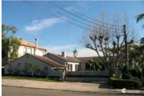
Figure 297 20 The Crescent, Vaucluse from the street
