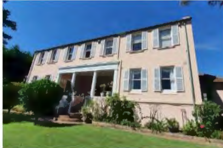
Figure 112 North elevation of 43 Latimer Road
