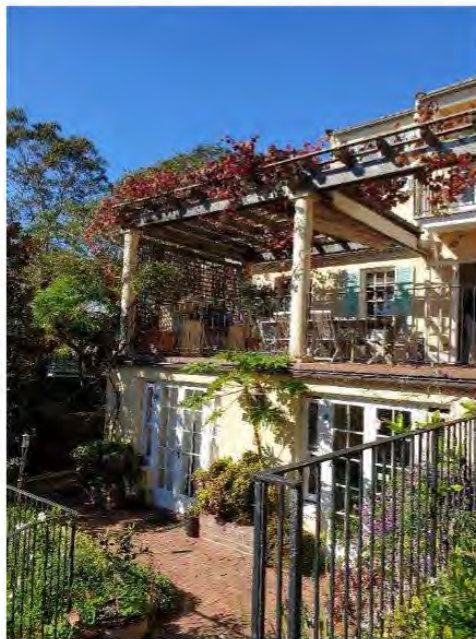
Figure 276 Pergola to the north elevation
